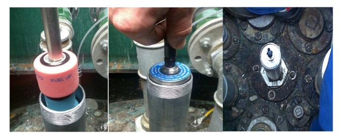
After positioning into the tank, tighten the PA antenna protection supplied with the probe;
