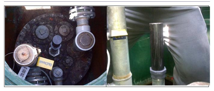
• Finally tighten the PA 2" protection supplied with the wireless probe applying a sealant product (Loctite, etc.) between the male riser and female, paying attention not to force too much the screwing.
