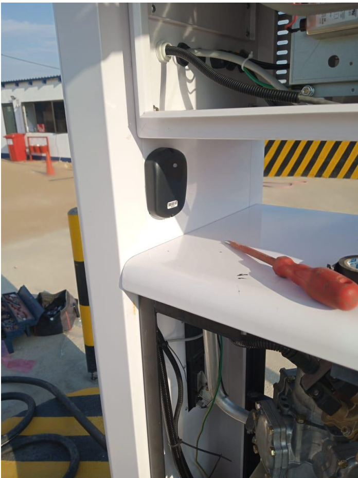
Example of reader installation on fuel dispensers
