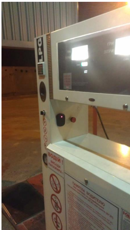
Example of VRD-E reader installation on fuel dispenser
